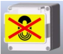
Prisma scan room quench button with plexiglass covers
