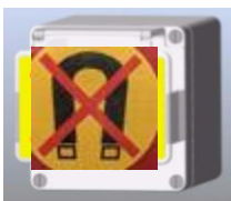
Prisma and mMR scan room quench button is behind the plexiglass cover
